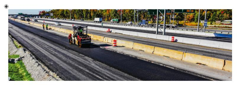
To make sure that the SEISMIC ASPHALT technology performs as expected, we have performed a series of trials and field tests. The trials were performed on various asphalt mix types and layer thicknesses. From the paved and compacted lanes, no less than 360 core samples
