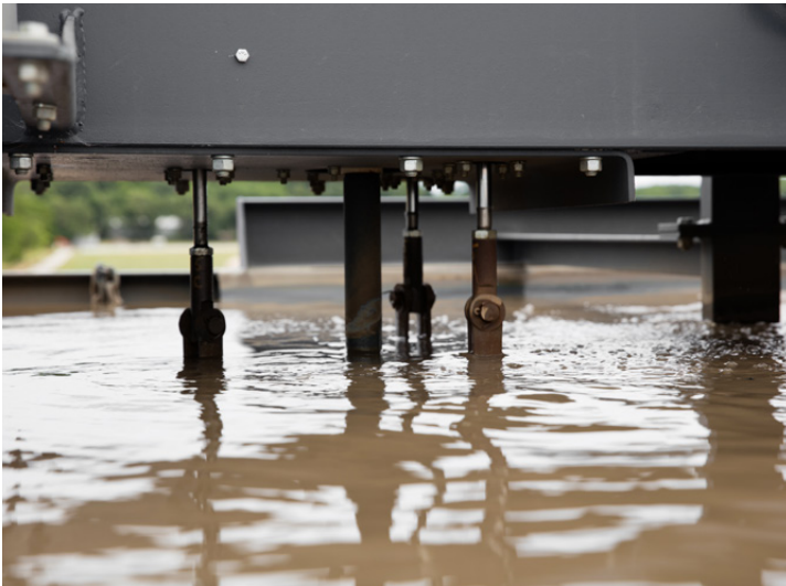
06/ FULL-LENGTH VALVE BRIDGE
