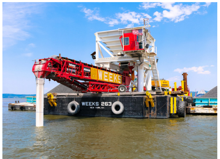
BARGE UNLOADING / DREDGE CAPPING
