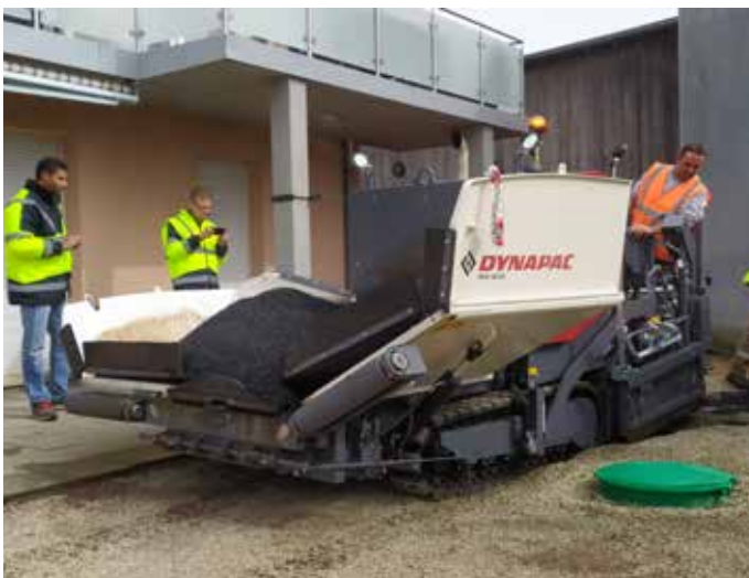
Paving in tight/narrow situations
