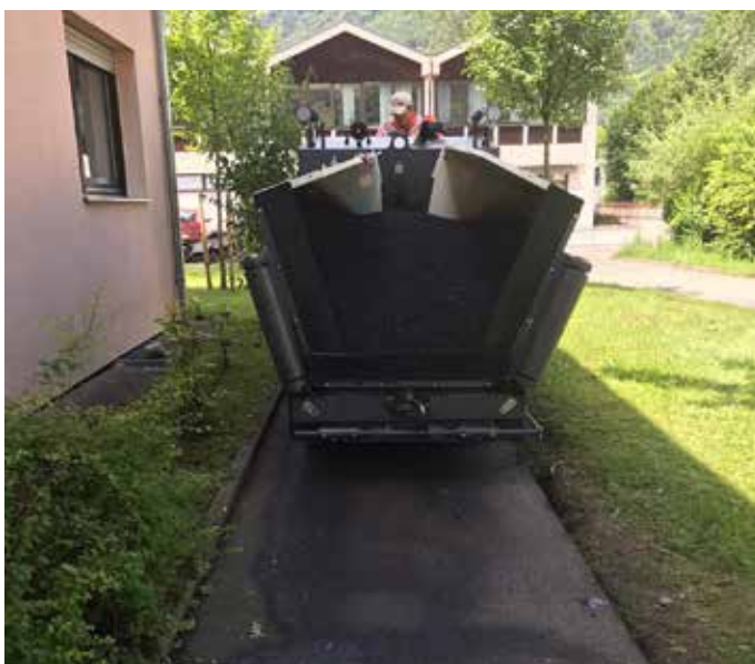
Paving bicycle path, trenches and side walks
