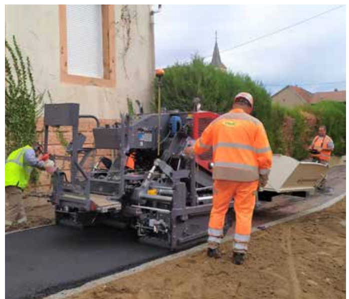
Paving and maintaining of city roads
